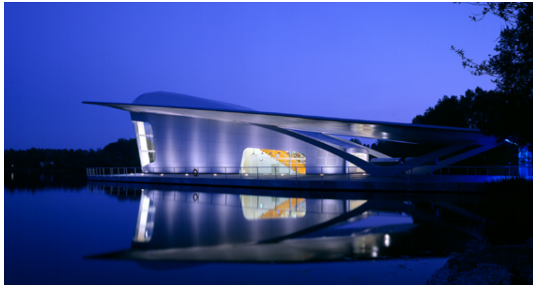
HydraPier Pavilion, Haarlemmermeer, The Netherlands
